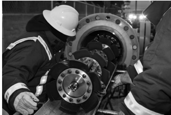
Figure 4. An in-line inspection (ILI) tool. Image used with permission, http://www.atcopipelines.com/upr/Media/
