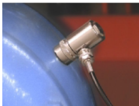
Figure 4. Installation of sensors
