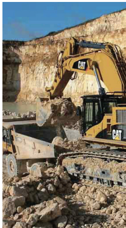
Figure 5. Heavy machines at work (from Caterpillar)
